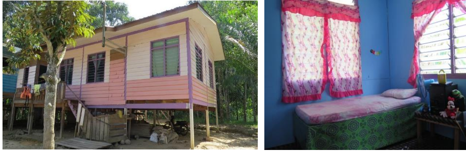
Figure 11-12: The renewed house to make homestay at Kampung Bahagia
