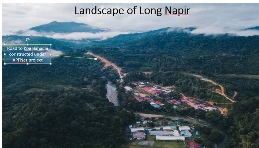
Figure 13: Road to Kpg Bahagia constructed under APFNet project
