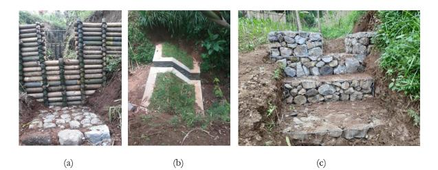
Figure 24. Types of gully control technique (a) Bamboo (b) Spesi (cemented stones); (c) Gabion
