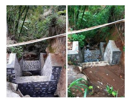
Figure 28. After small check dam was completed (a), it collected sediment (b)
