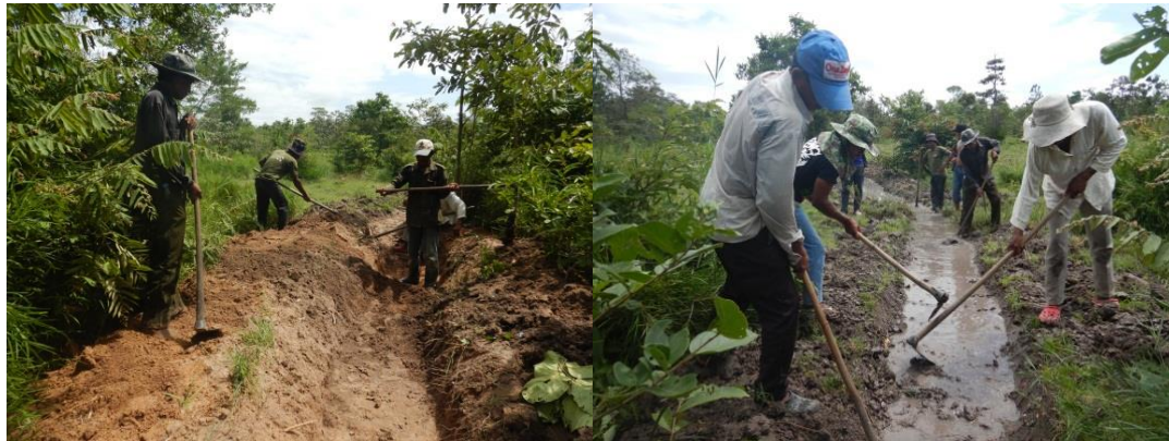
Figure 18. Drainage canal constructed in the restoration site
