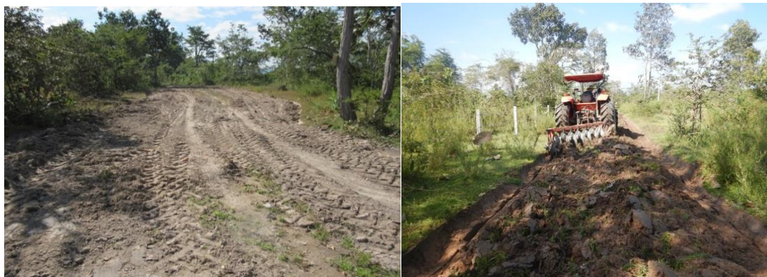
Figure 19. Fireline constructed around the project site
