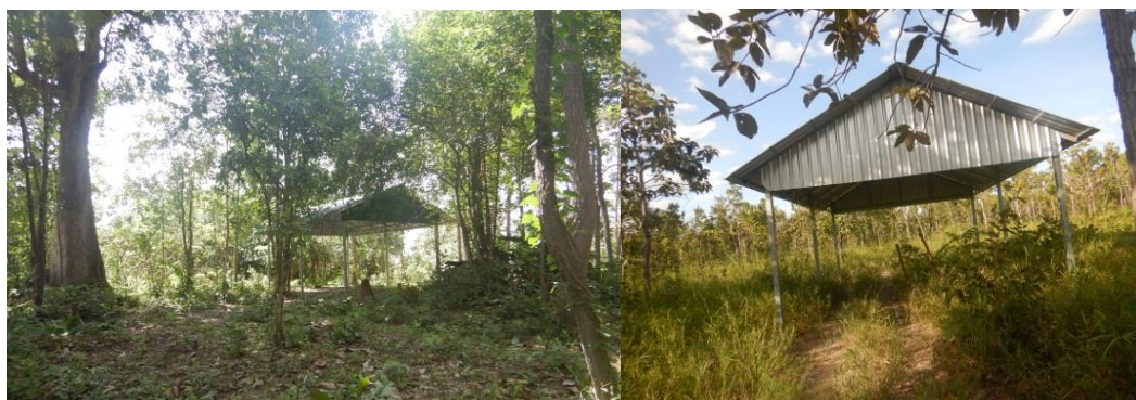
Figure 6. Constructed guard house for the CF Patrol Team
