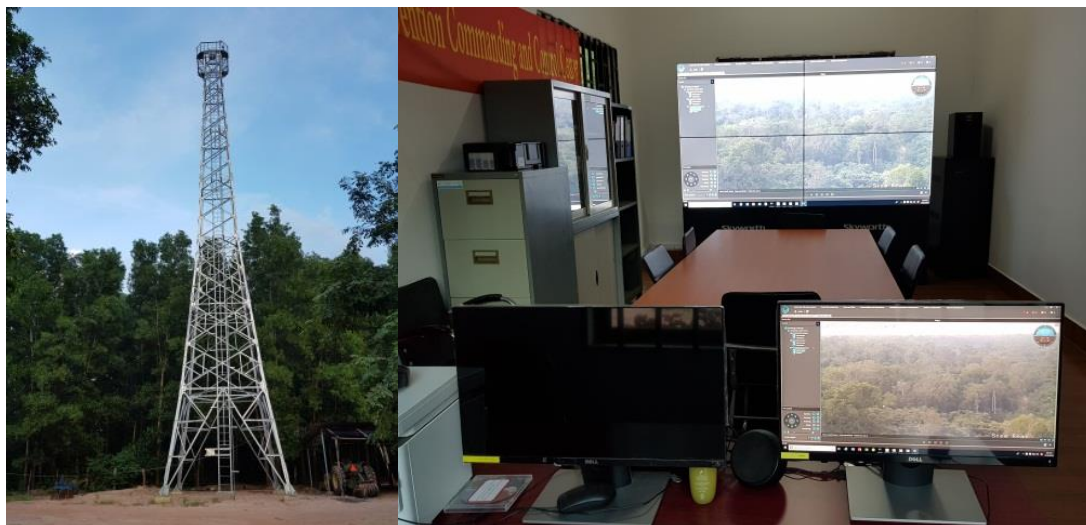
Figure 34. Forest Watcher tower (left) and the monitors in the office
