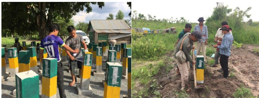
Figure 4. Production and installation of the corner posts
