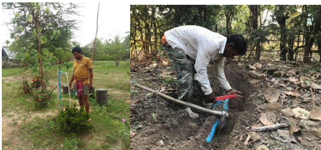
Figure 26. The CF members conducting repair of the pipe system
