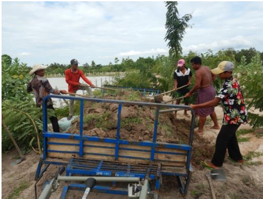
Figure 23. CF members stabilizing the dikes of the water pump
