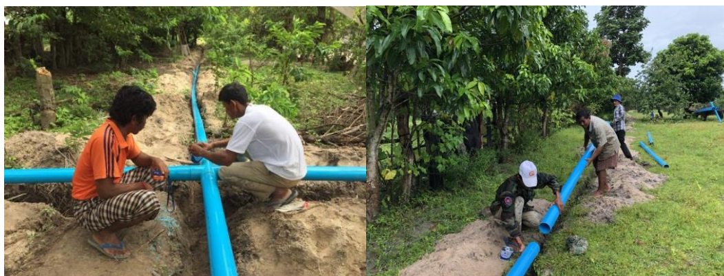
Figure 25. CF members laying out the water pipes
