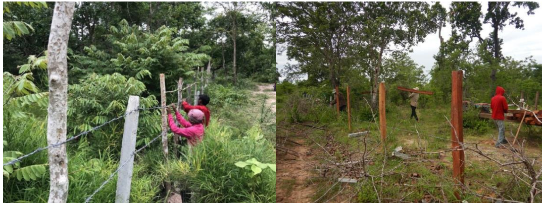
Figure 20. CF members repairing the fence
